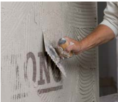
Ytong Armeringsnett glattes 1/3 inn i grunnpussen.
